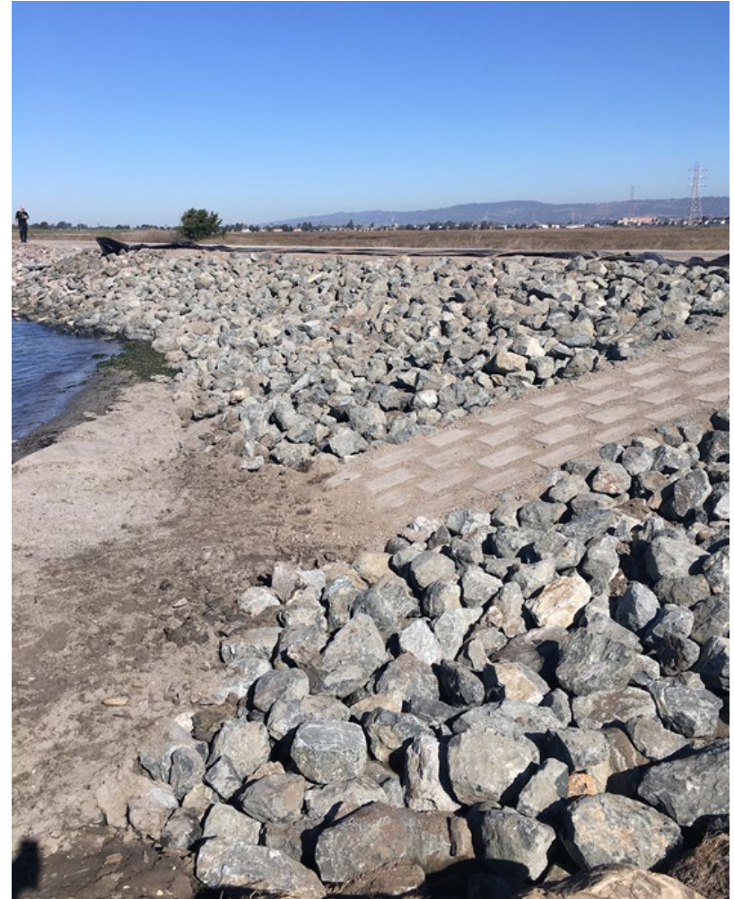
COMPLETED WORK WITH ENGINEERED LEVEE
